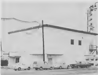
Oil Movements Control Center regulates flow of all crude and crude products by computer.
